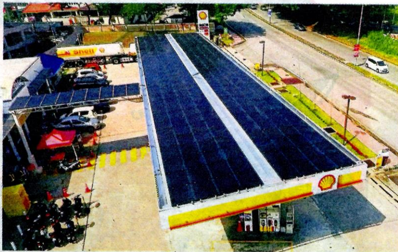
▲ An aerial view showing the solar panels on Shell's Damansara Jaya station.
